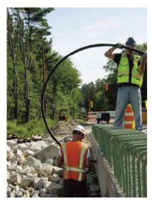
Passing CFCC strand through duct Fig. 10—Little Pond Bridge.
