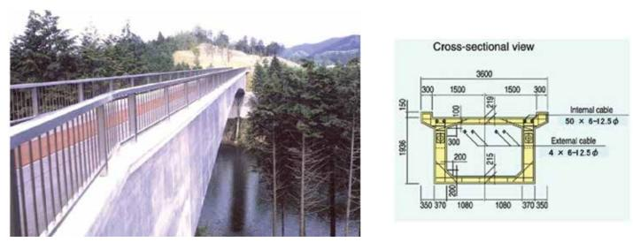
Fig. 4—Hisho bridge side view and cross-sectional view. (Note: All dimensions in mm; 1 in. = 25.4 mm.)
