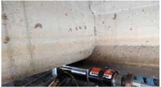
Post-tensioning cable with load cell Fig. 12—I-10 New Orleans East Girder Repairs, Louisiana.
