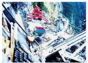
Easy handling at the narrow space Fig. 16—Installation of new ground anchor system using CFCC.
