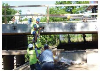
Passing CFCC strand through a duct Fig. 9—M-50/US-127 Highway over Norfolk Southern Railroad.
